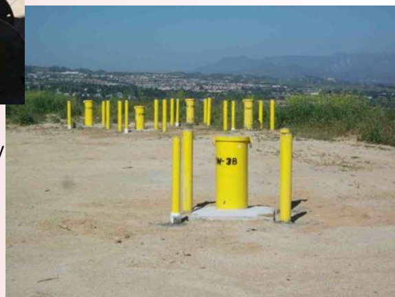
Below: Completed extraction well with piezometers in the background.
