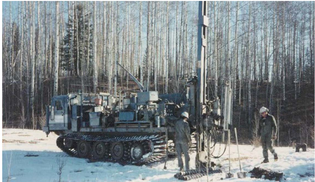
Photo courtesy Great West Drilling
