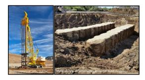
The deep mixing method increases the strength and decreases the compressibility of soft ground, and thereby improves stability and reduces settlement of embankments, including transportation embankments, MSE retaining walls, levees, and dams. Continuous shear panels oriented perpendicular to the embankment alignment are more efficient for stability than isolated columns because shear panels are not subject to the same
